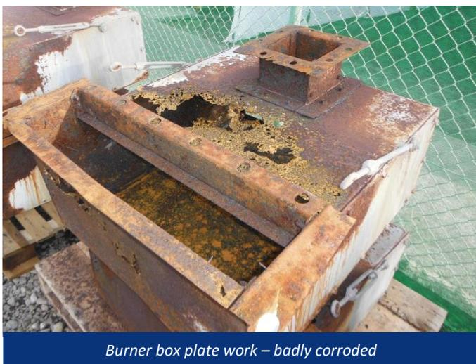
*Burner box plate work – badly corroded*
