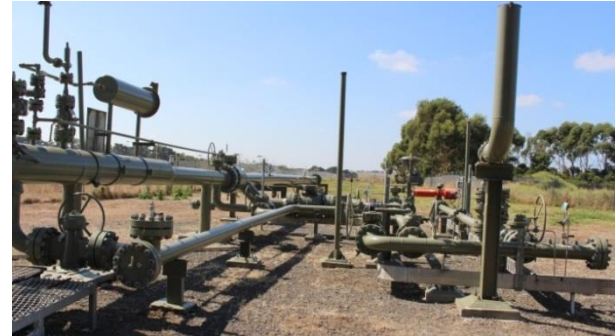
North Paaratte – Pig Launcher Upgrade - BEFORE
