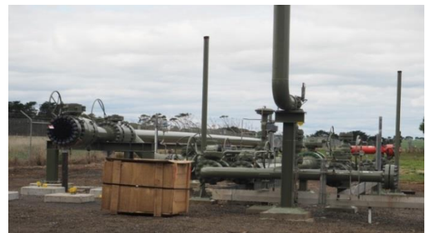
North Paaratte – Pig Launcher Upgrade - AFTER
